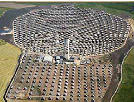
A 'power tower' type of CSP plant near Seville, Spain; photo credit: Abengoa
